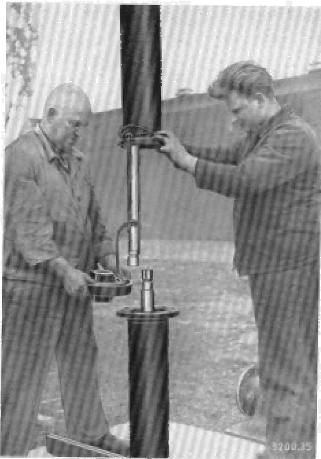
Fig.17 – Rising main with suspended shaft
